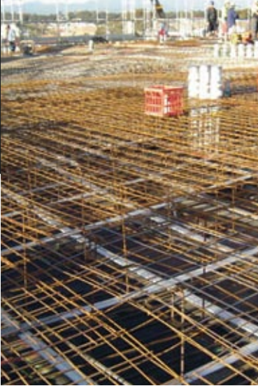
Level 6 post-tensioned transfer floor
