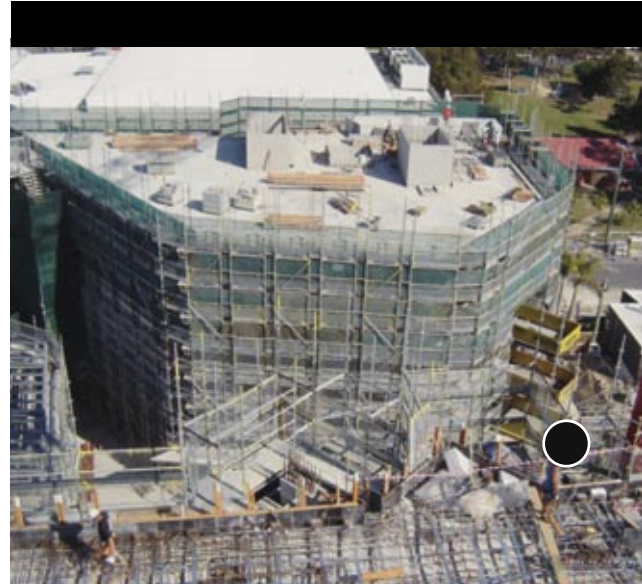
Tower 1 under construction
