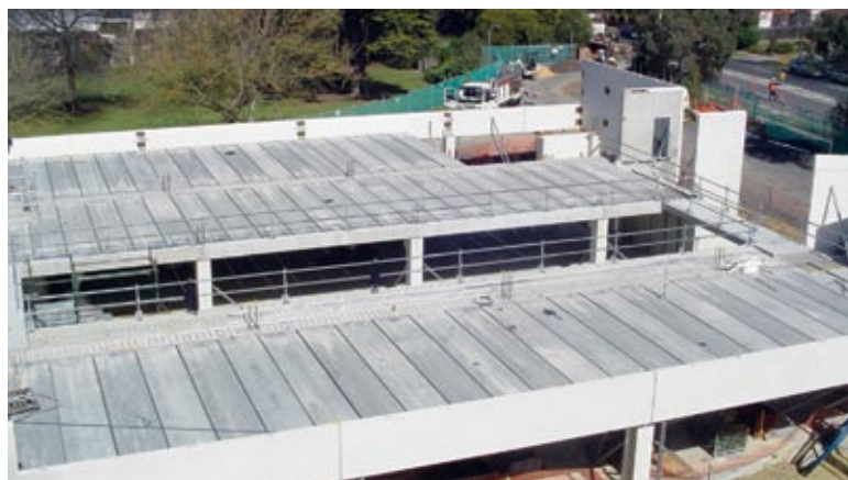
Long spanning precast hollow-core floor planks prior to concrete topping
