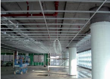
Fit-out follows closely behind construction
