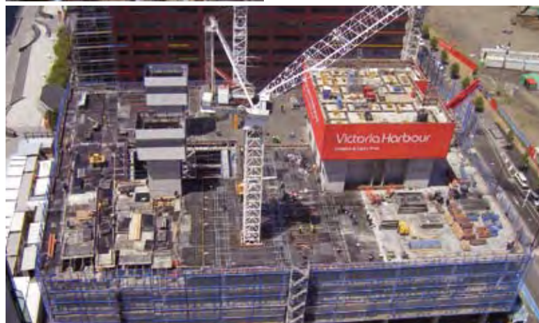
below: Aerial view showing the large floor plates under construction
