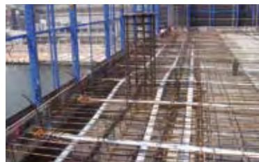
left: Detailing of post-tensioned perimeter beams
