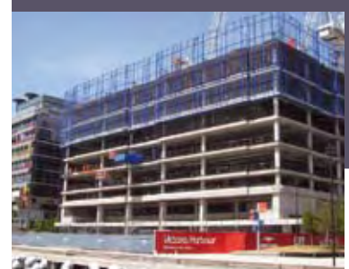
North east elevation showing the concrete framed structure under construction
