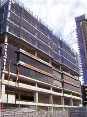
Movement sensitive facade system is supported by post-tensioned concrete perimeter beams
