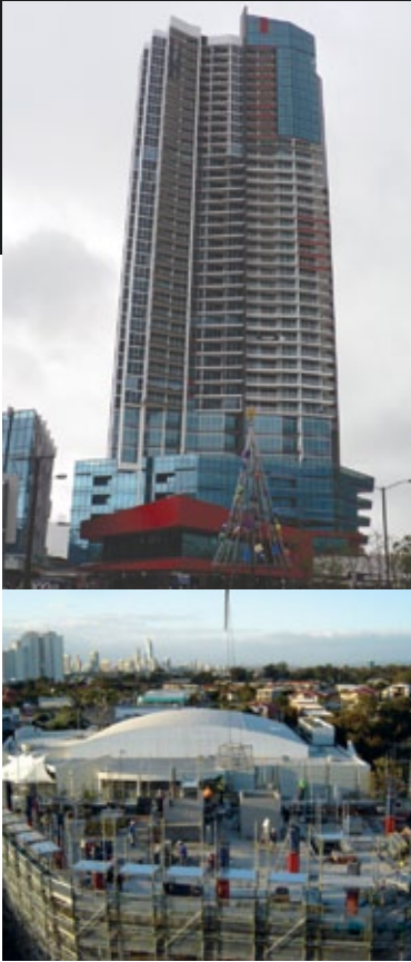
Precast columns shown on 40 storey Southport Central, Queensland
