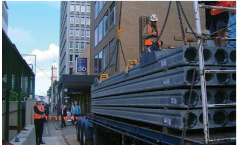
Precast hollowcore floor planks arriving on site, Santos office building, Adelaide
