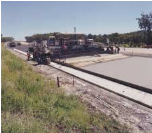
Figure 1 View of slipform paving machinery
