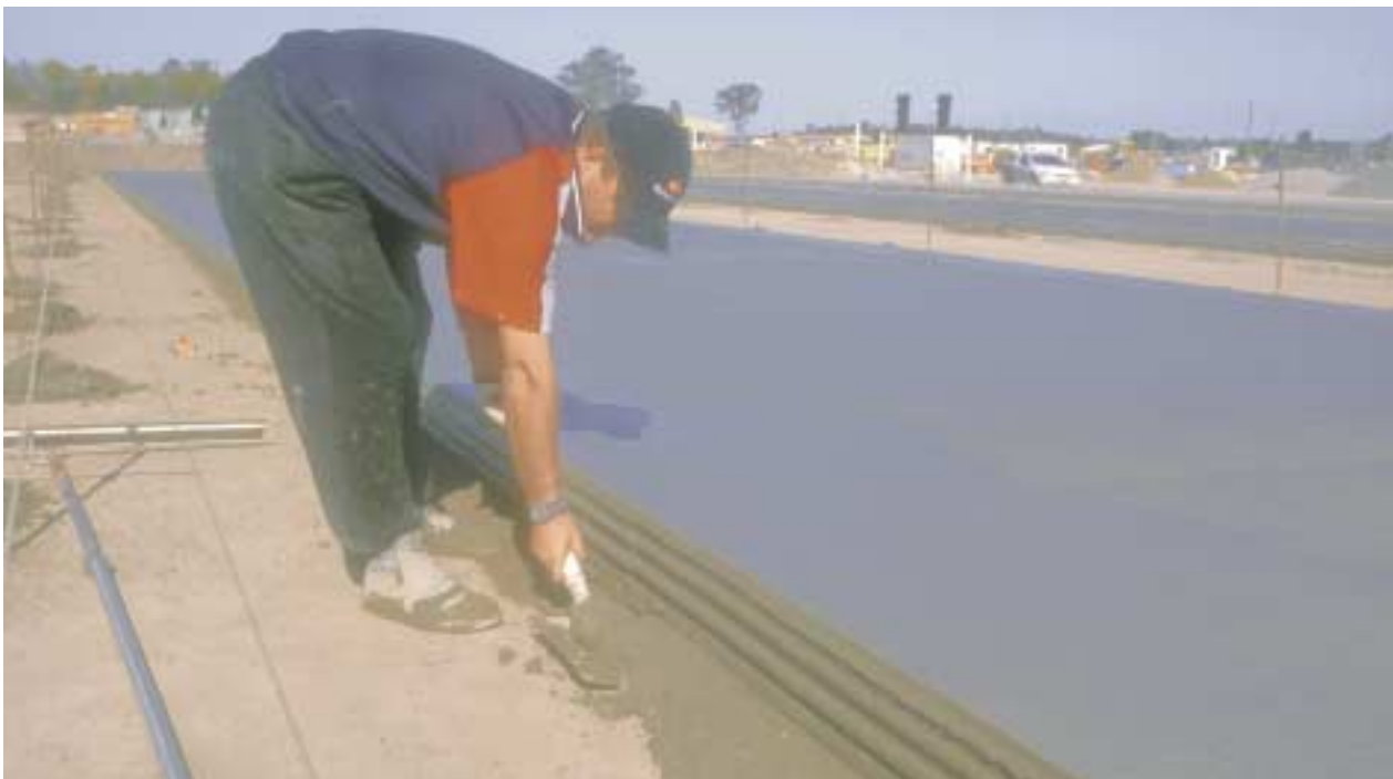
Figure 3: Corrugated profile for longitudinal joints
