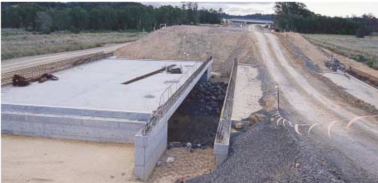
Figure 10: Typical motorway bridges with additional surcharge on approach transition zones
