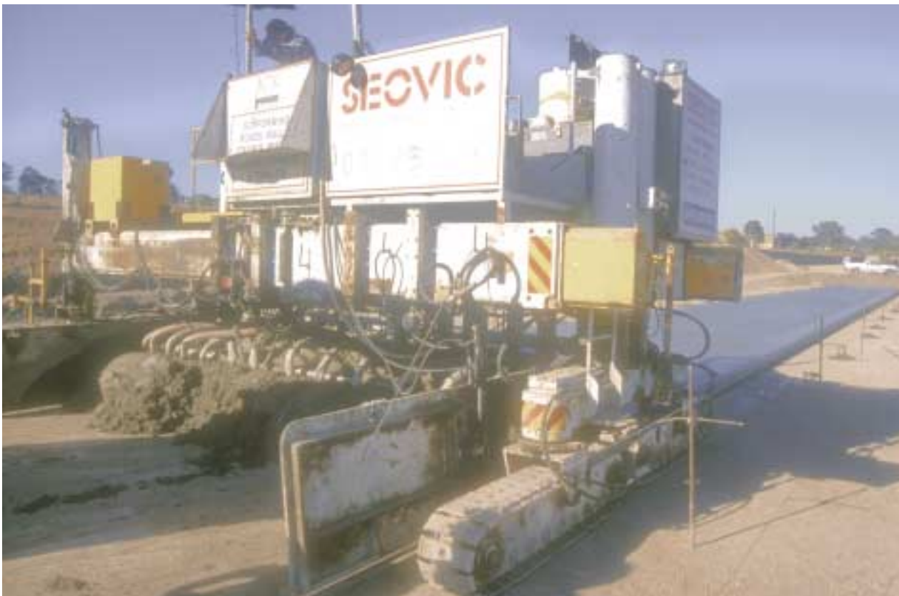
Figure 1: M9000 slipform paver floor levels set using string line
