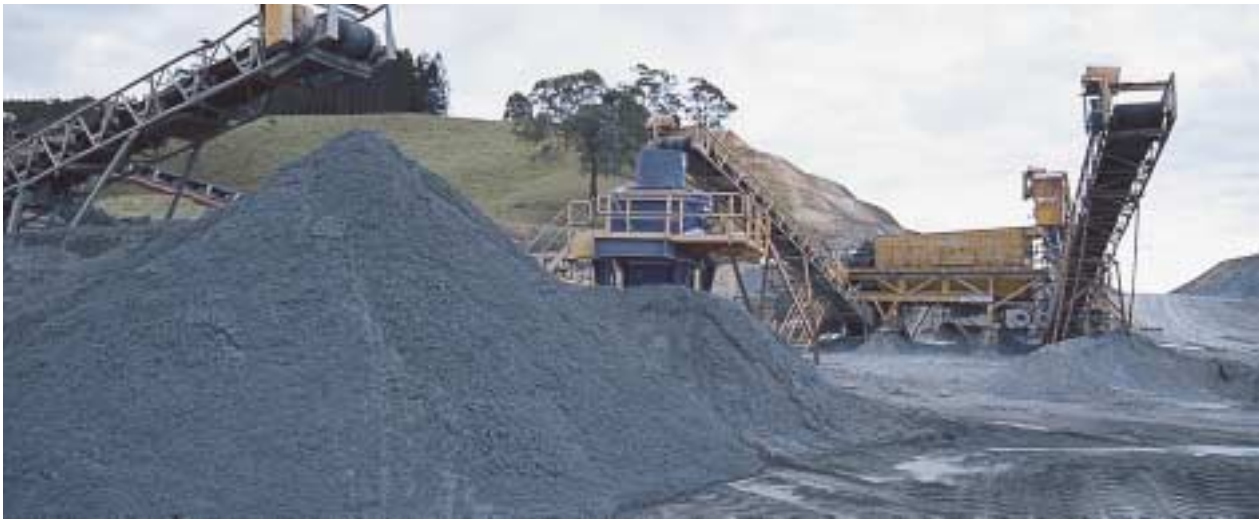
Figure 7: Manufactured sand stockpile and crushing plant
