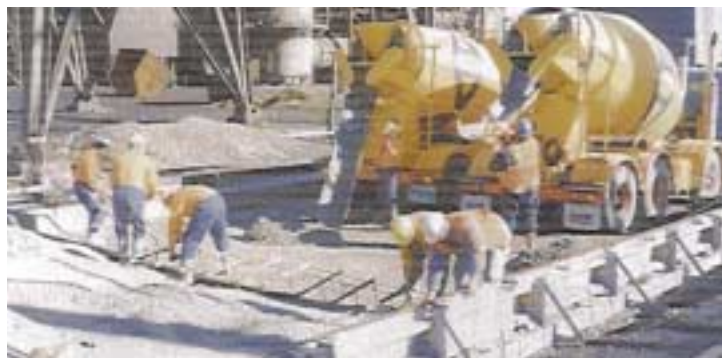
Figure 3: Placing the dowel bars for the expansion joint
