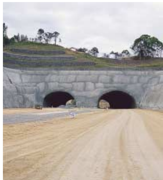
Figure 9: Cudgen Road tunnels
