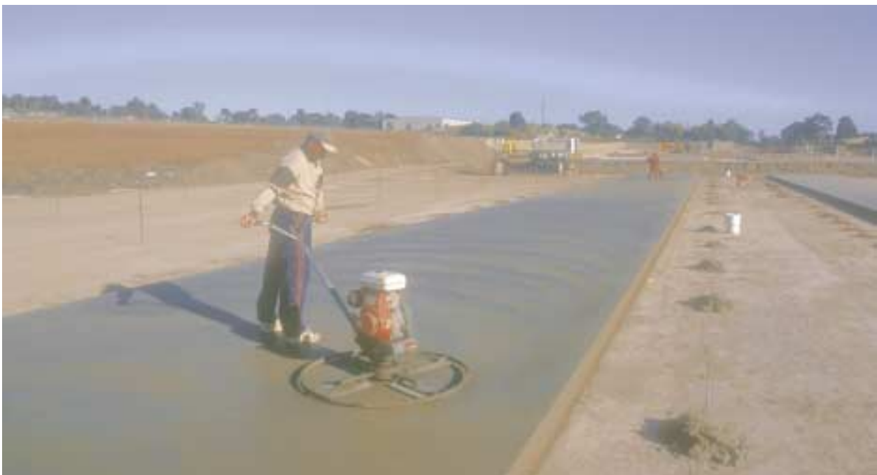
Figure 5: Surface is power trowelled
