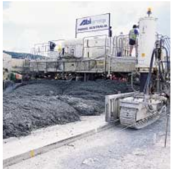
Figure 5: Paving the 8-m wide section of the base
