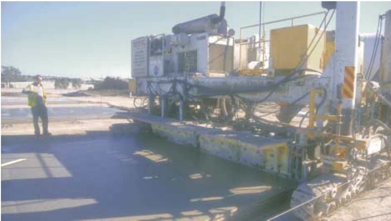
Figure 2: Screed plate ensures compact surface and level tolerances
