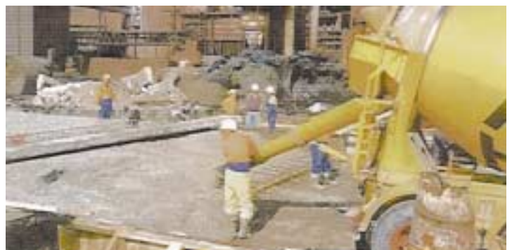
Figure 4: Pouring concrete on Road 30
