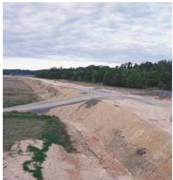
Figure 2: Formation constructed on unconsolidated marine silts
