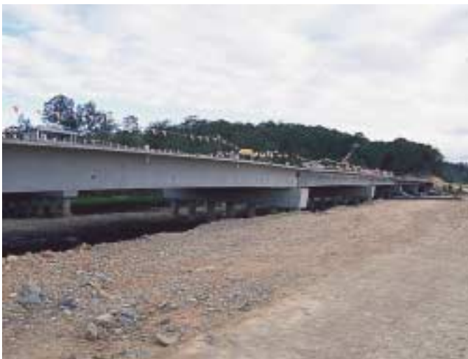
Figure 4: Precast concrete bridge across floodplain
