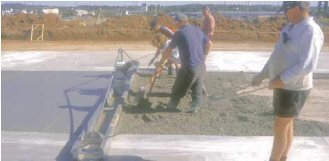
Figure 6: Intermediate slabs are placed using a vibrating screed
