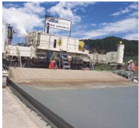
Figure 6: Hessian-drag finish to surface
