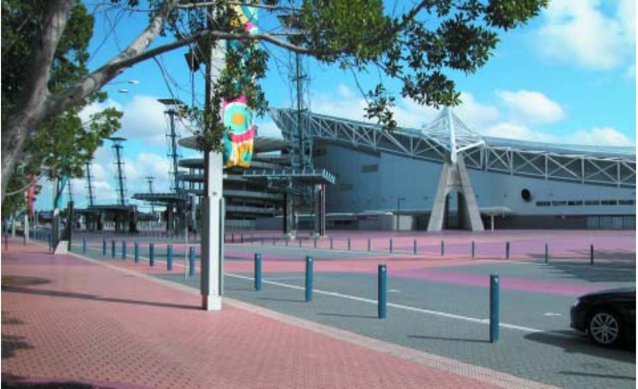
Segmental paver colours provide delineation for vehicular and pedestrian movements
