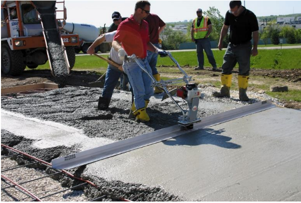
Figure 12.18 – Vibrating Screed in Use 12.9
