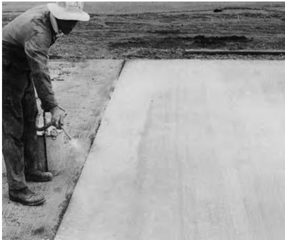
Figure 15.8 – Spray Application of Curing Compound
