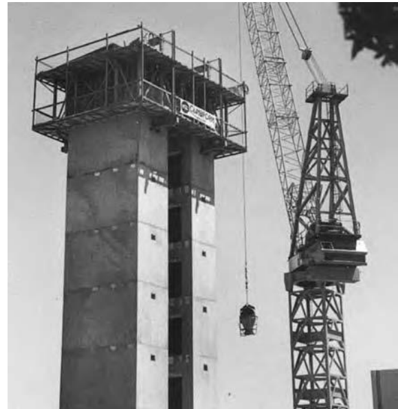
Figure 27.8 – Typical Self-climbing Formwork System
