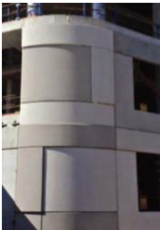
Figure 20.11 – Precast Cladding Wall Panels
