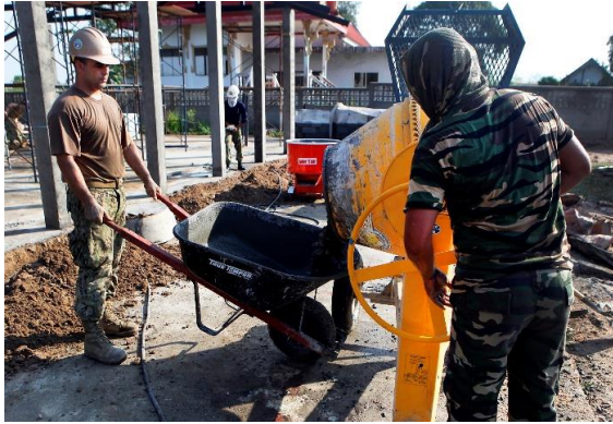
Figure 12.5 – Barrows, despite their limitations, are the Most Suitable Distribution Means on Small Projects 12.2
