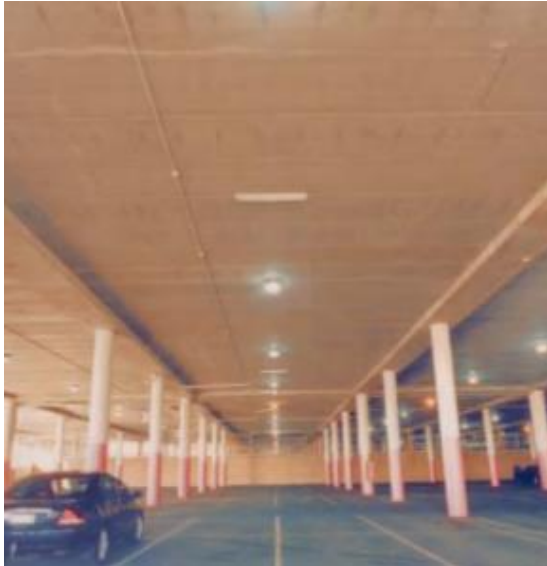
Figure 20.19 – Long Span Hollowcore Flooring provides Space during Construction and Use
