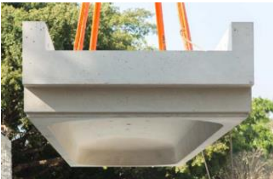
Figure 23.2 – 'Geopolymer' Precast Floor Panels used in Global Change Institute, University of QLD
