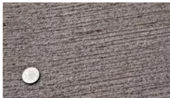
Figure 14.7 – Broom Finishing helps to provide Skid Resistance
