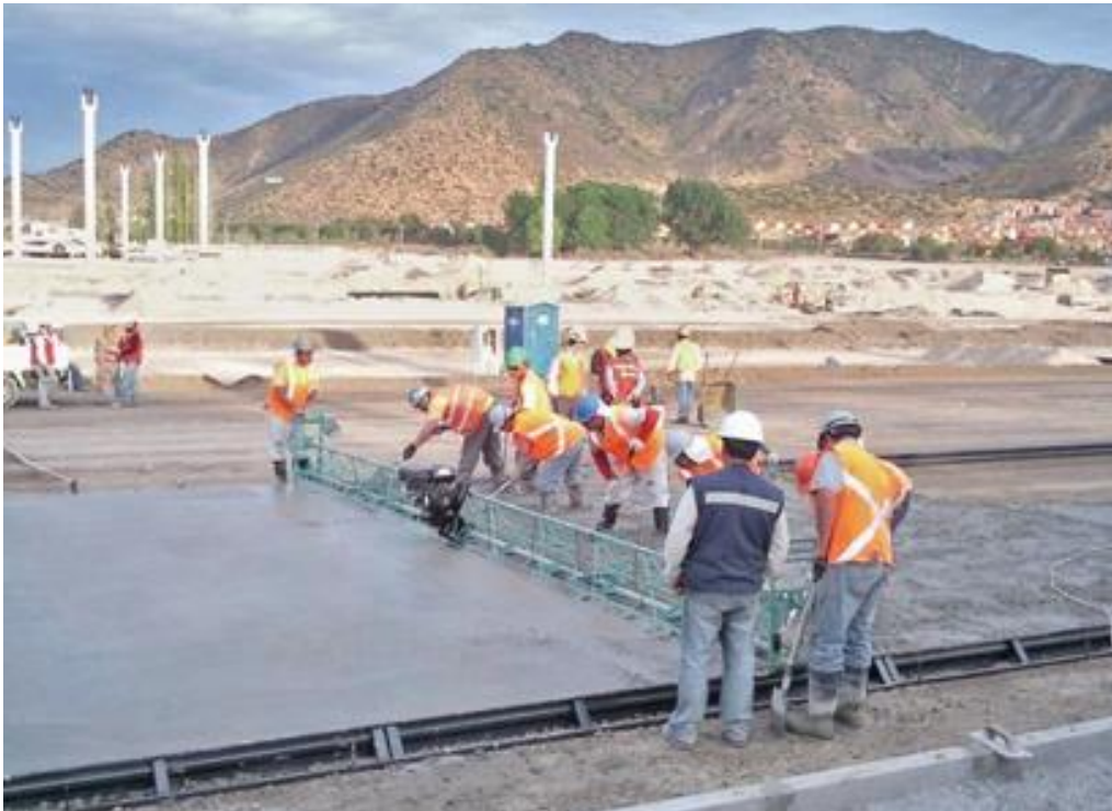
Figure 14.1 – Typical Trussed Vibrating Beam Screed
