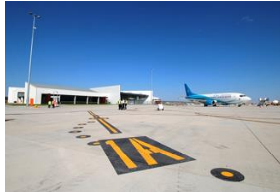
Figure 23.3 – 'Geopolymer' Concrete Use – Aircraft Pavement and General Building – Wellcamp Airport
