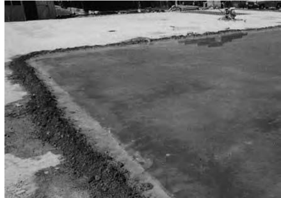
Figure 15.9 – Ponding Method of Water Curing
