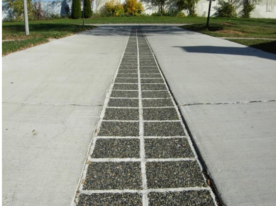
Figure 24.2 – Porous Concrete Pavement in the Middle Strip of Two Parallel Concrete Pavements 24.2
