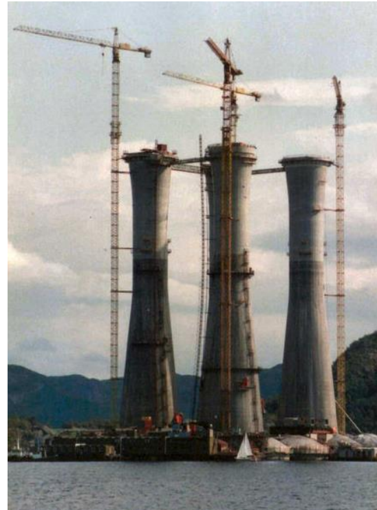
Figure 19.3 – Tapered Slip-forming 19.1
