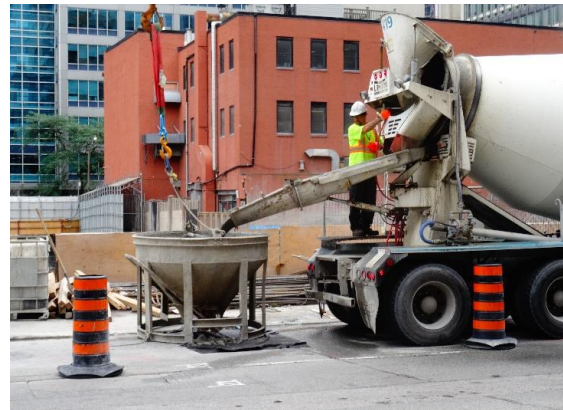
Figure 12.7 – Crane Buckets and 'Kibbles' are easily filled from Transit Mixers 12.3
