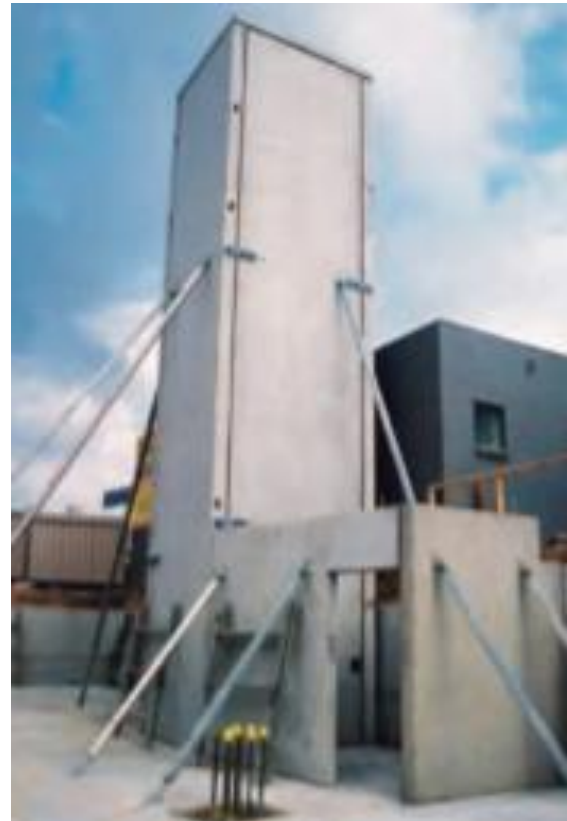
Figure 20.14 – Precast Wall for a Lift Shaft and Stair Core
