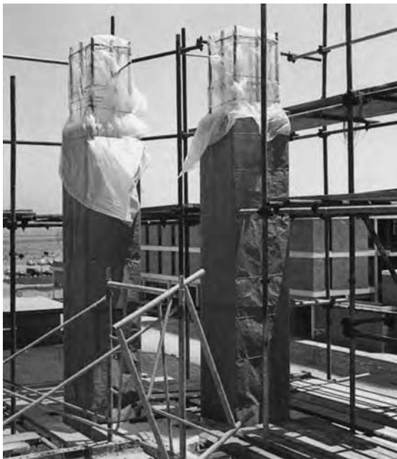
Figure 16.9 – Completed Work and Reinforcement protected by Wrapping
