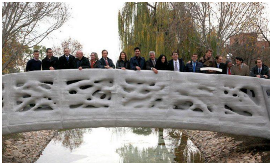
Figure 24.10 – 3-D Printed Bridge, Powder-based Technique 24.10
