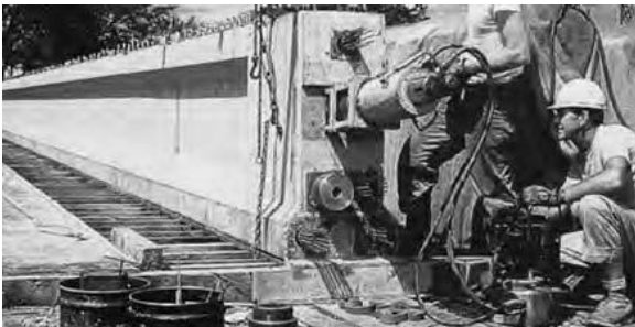
Figure 1.25 – Post-Tensioning Jack Operating at an End of a Concrete Girder
