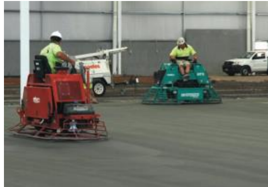
Figure 14.6 – Multi-head power Trowel Machines are commonly used for Major Warehouse Projects
