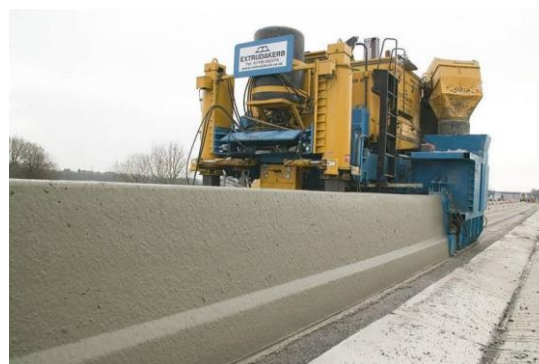
Figure 19.9 – Barrier Wall Under Construction 19.4
