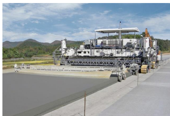
Figure 10.2 – Concrete Paving using a 'Slip-form' machine 10.1
