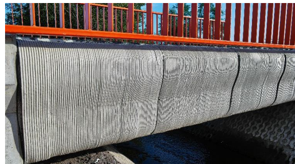
Figure 24.9 – 3-D Printed Bridge, Extrusion-based Technique 24.9
