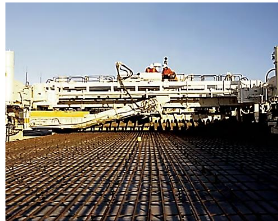
Figure 19.6 – Paving Machine and a CRCP Pavement
