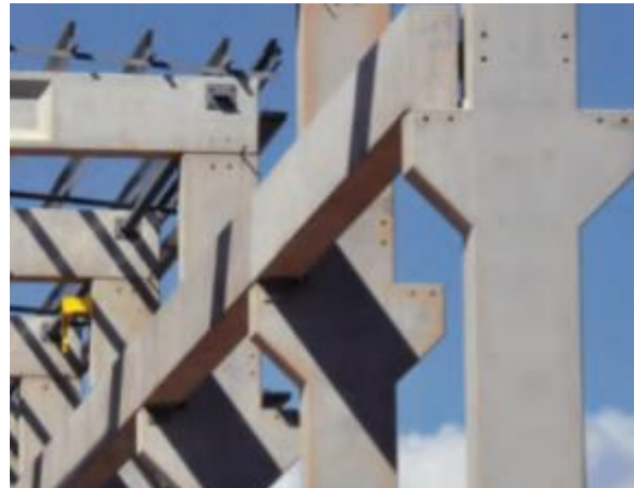
Figure 20.10 – Precast Concrete Columns supporting Structural Beams
