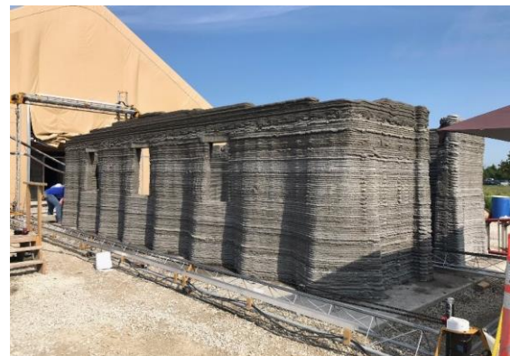
Figure 24.8 – 3-D Printed House, Extrusion-based Technique 24.8
