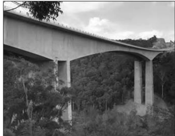
Figure 11.7 – Multi-strand, Post-tensioned bridge, Mooney Mooney, NSW
