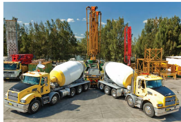
Figure 10.1 – Truck Mounted Transit Mixers delivering Concrete to a Pump on Site
