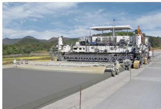
Figure 10.2 – Concrete Paving using a 'Slip-form' machine 10.1
