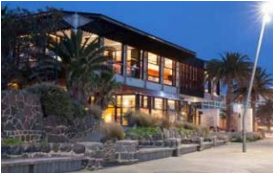
Figure 23.4 – The Stokehouse (Melbourne) was constructed using Envisia TM Concrete
