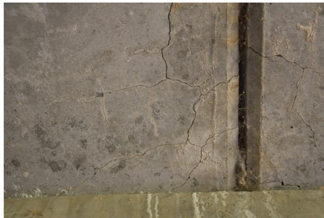
**Figure 1. Cracking of bridge beams due to ASR**
