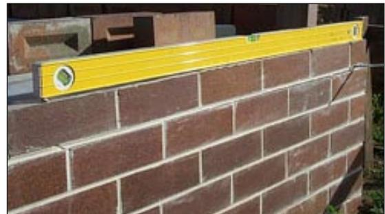
**Figure 2:** Curling of infill slab corner, lifting the brickwork bonded to it.
