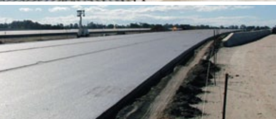
Figure 3 Sydney's Westlink M7 motorway, a continuously reinforced concrete road pavement 8
