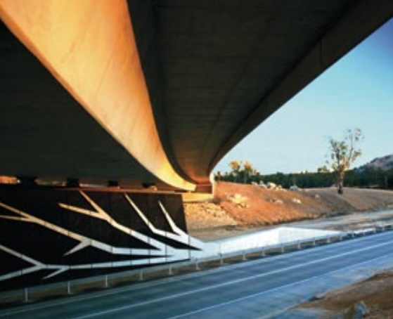
Figure 1 Tumbarumba Bridge, Wagga Wagga NSW (winner of the bridges category, 2009 Public Domain Awards)
