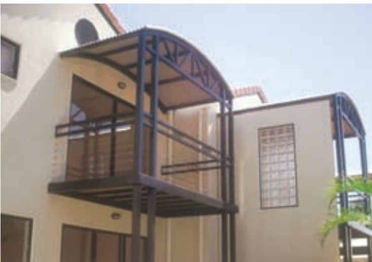
Simple features can produce an interesting facade
