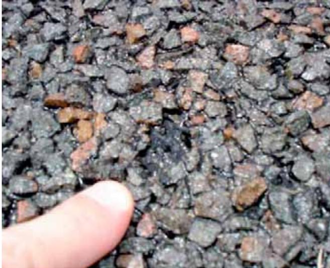
**Figure 8: The commencement of aggregate stripping from a pavement surface**
