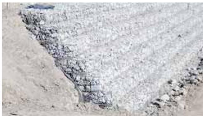
Figure 2: Typical gabion wall application
