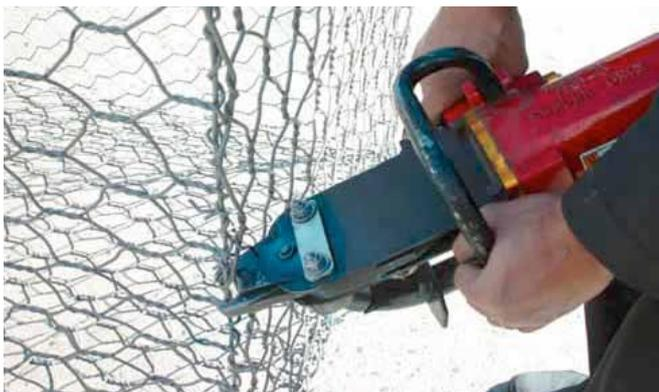
**Figure 5B: The lacing process**
