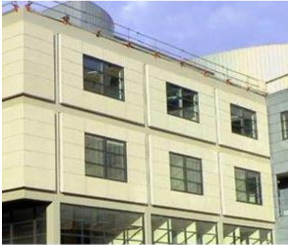
Figure 4: Concrete frame may require tolerances appropriate for the fitting of components such as precast units.
