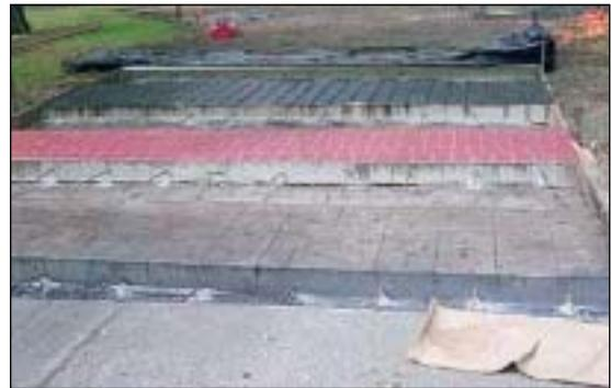
**Figure 3:** The concrete pavement was placed in two stages with dowel bars along all construction joints
