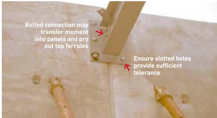
**Figure 16: Panel/Rafter connection - not recommended**
