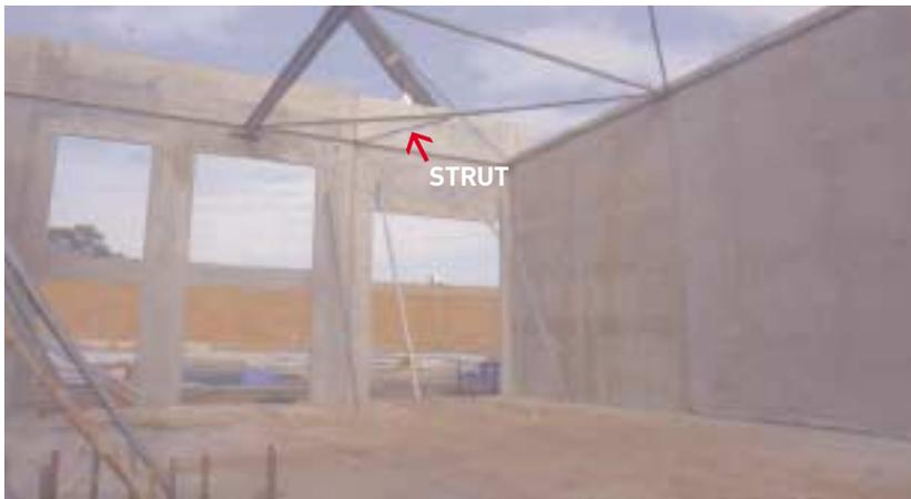
Figure 14: Rafter to panel connection at joint
